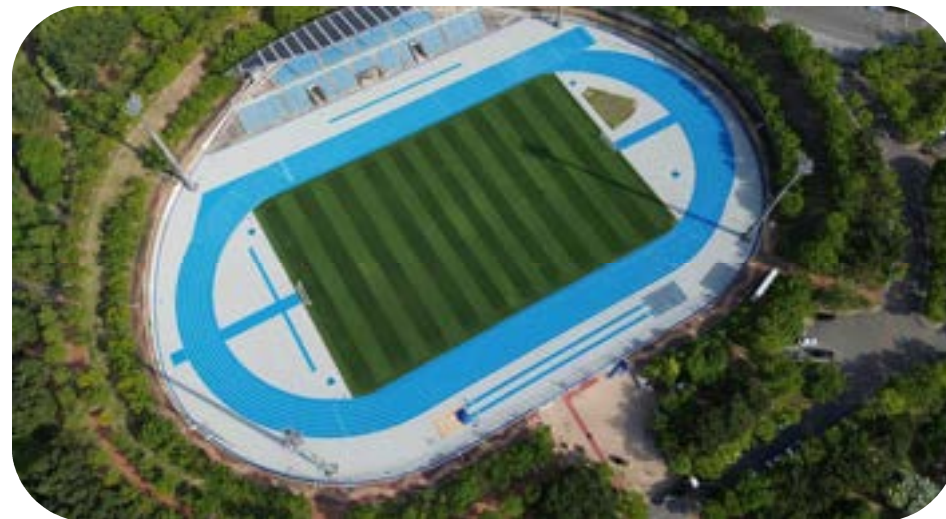
<Daegu Auxiliary Stadium - Inside View>
